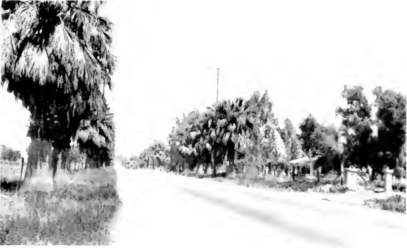
FIGURE 2. THE SOUTHERN TRANSCONTINENTAL ROUTE NEAR PHOENIX, ARIZONA.
